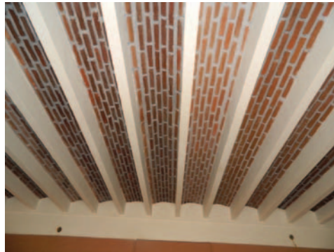
Fig. 15. Madras terrace (ground floor)
