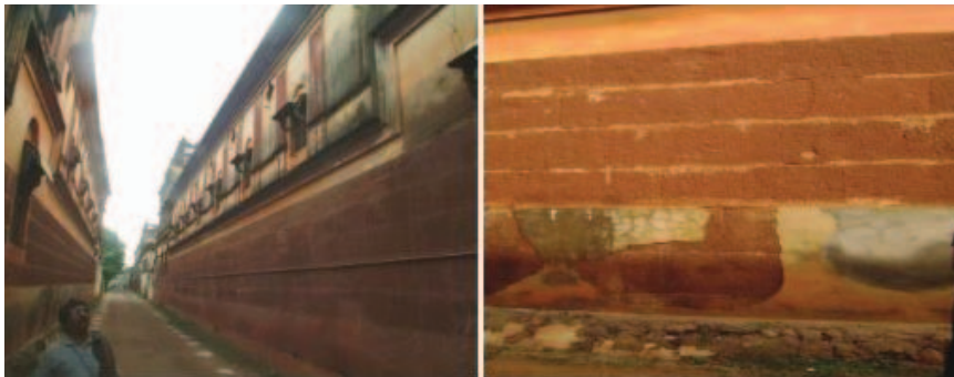
External wall plastering
