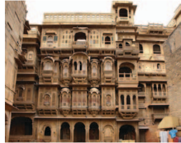
Vertical air shafts
