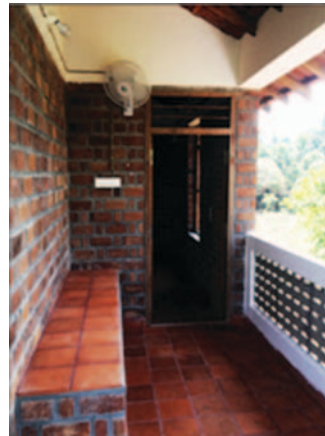
Fig. 29 Sit out (first floor)
