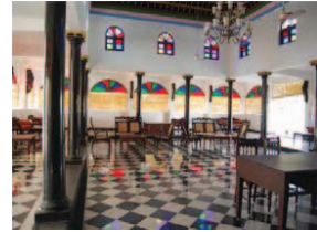
clear storey windows
