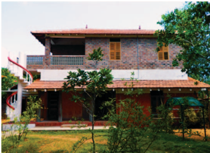
Fig. 26 View of cottage
