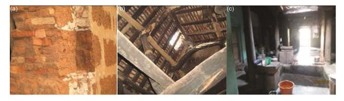
Fig. 6—Building components and construction techniques: (a) Flat brick wall with laterite block covering (b) Naturally processed wooden roof trusses (c) Courtyard at the centre aligned along the axis
